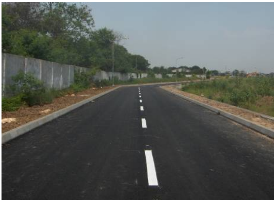
Access Road – After one year of maintenance period
