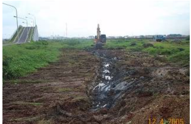
Existing Condition of the Inspection Road
