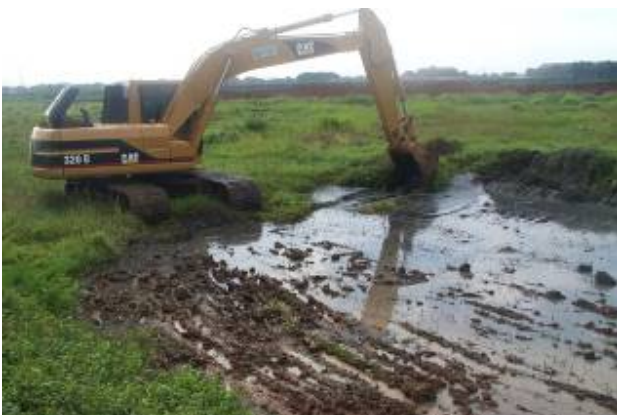
Dewatering & Land Preparation
