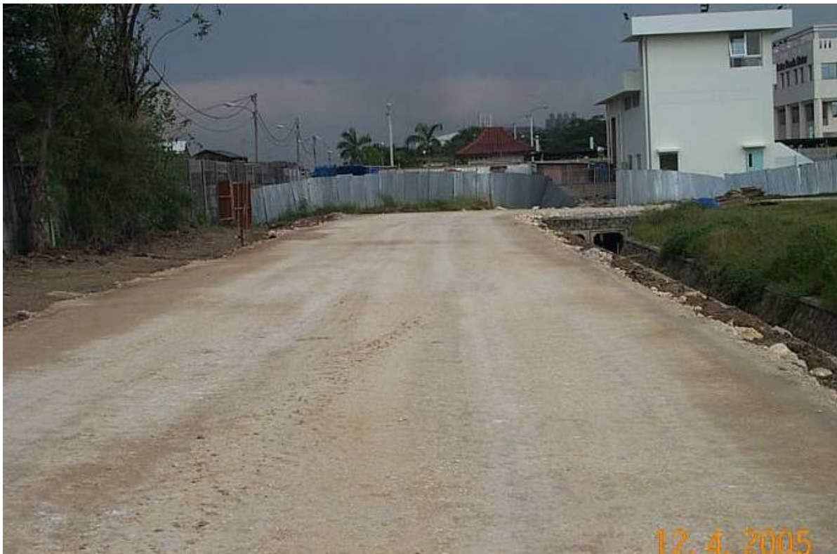
Pavement Structure Strengthening using Modified Cement Treated Base
