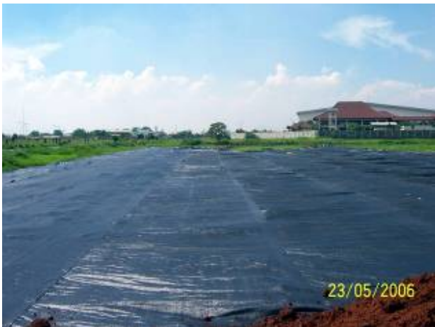
Soil Stabilization using geosynthetic 2 nd Stage Test Course
