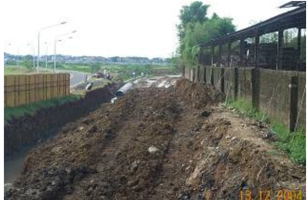
Existing Condition of the Access Road
