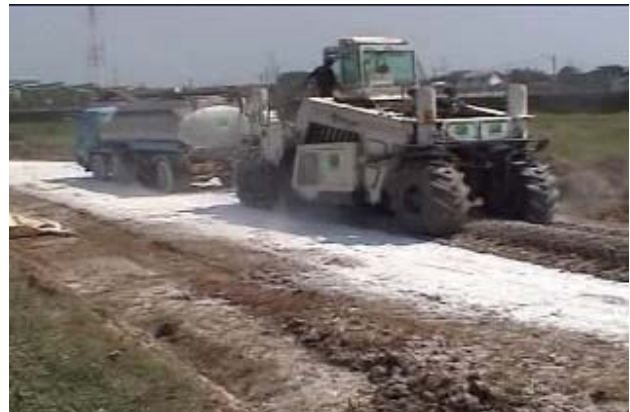
Soil stabilization using Hydrated Lime connected to a Water Tank
