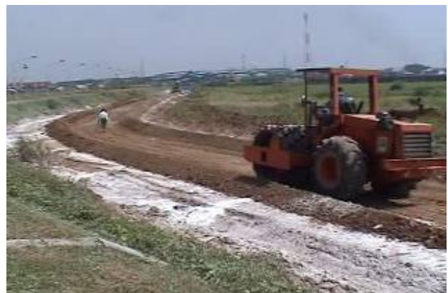
Trimming and Compaction
